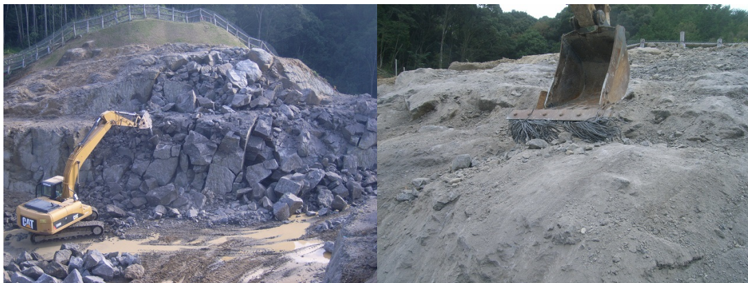
Figure 12. Careful finishing by heavy machinery at the secondary excavation
