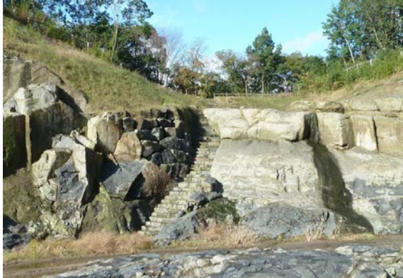
Figure 13. Steps placed between bedrock and stone walls
