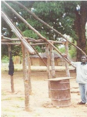
Figure 6. Construction system – Skeleton with pinpoints, Dipuduhudu, Botswana
