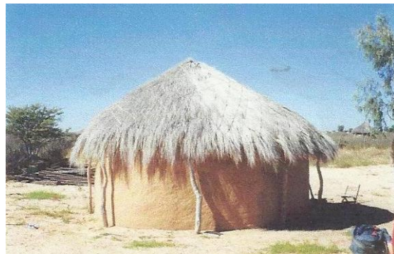
Figure 5. Finished traditional house at Dipuduhudu, near Molepolole, Botswana
