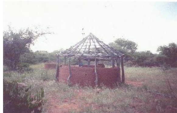
Figure 2. Partly finished house with visible construction system, Dipuduhudu, Botswana
