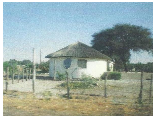
Figure 12. Contemporary round house with solid structural walls and a thatch roof, Gumare
