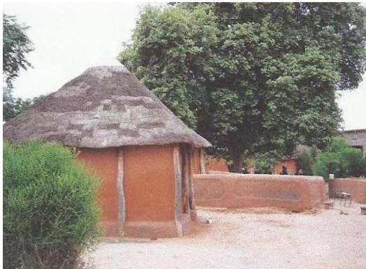
Figure 11. Contemporary square house with a thatch roof and a skeleton construction system, Serowe, Botswana
