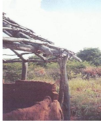
Figure 7. Traditional house – Details of the construction system
