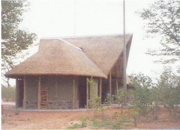
Figure 9. DWNP, Park Entrance Gate at Chobe National Park
